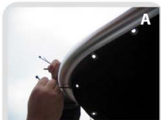
Temporarily fasten fabric to frame by wire tie or rope.
